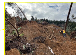
The landslide mass is riding up.
