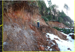
Main scarp (H= 5m)
