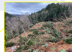
Many of the trees have fallen on the down slope side.
