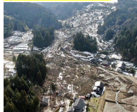
Fig. panoramic view of the landslide
