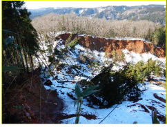
Main scarp (H=5~25m)
